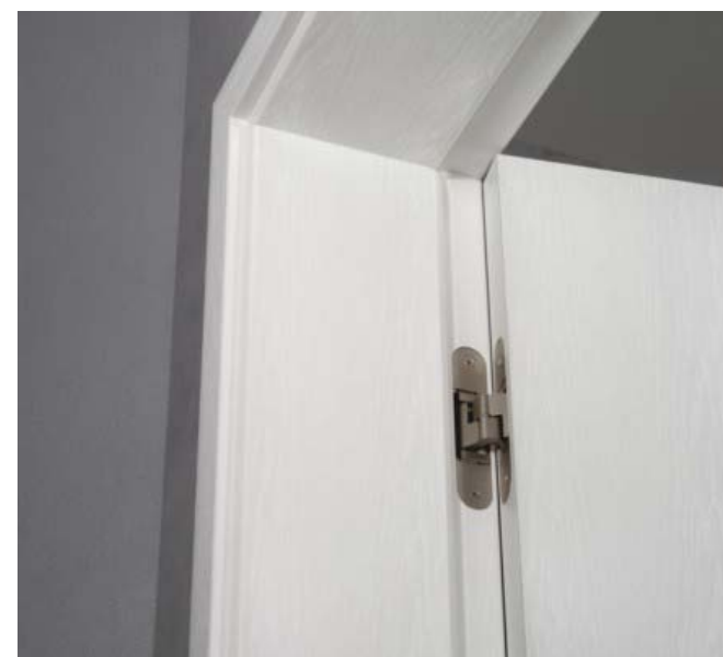
hinges are assembled in door and frame
