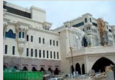
International Medical Center, Jeddah, Saudi Arabia
