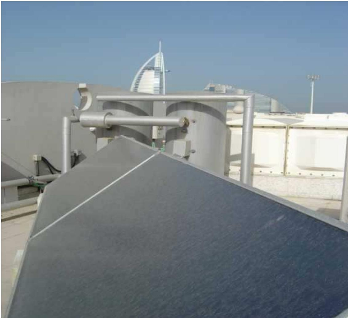
Solar hot water system with electric backup
