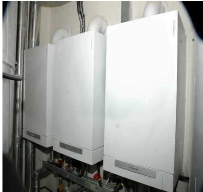
Viessmann Gas condensing boilers for the backup of the system (109 % efficiency)
