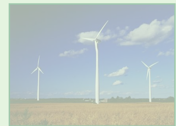
Wind Power Generation
