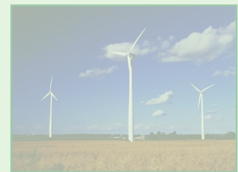
Wind Power Generation
