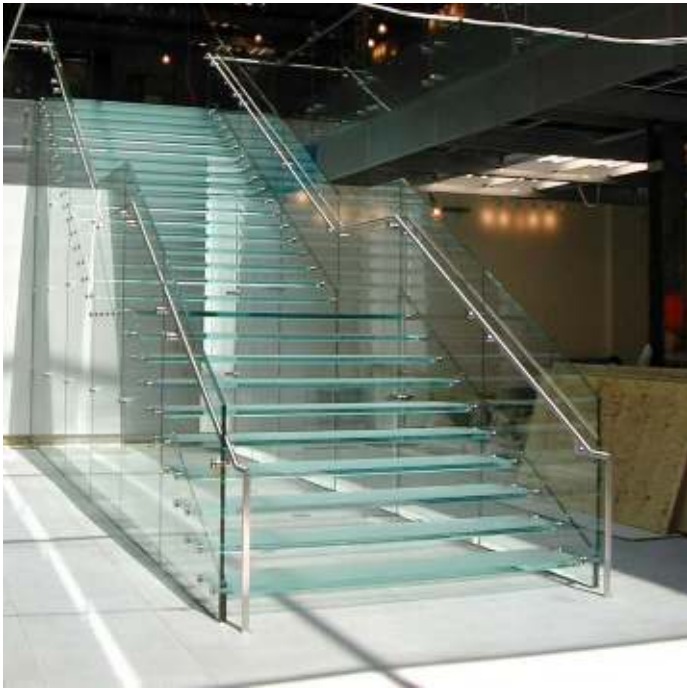
Laminated glass, stair treads and bridge at Apple Store, New York
