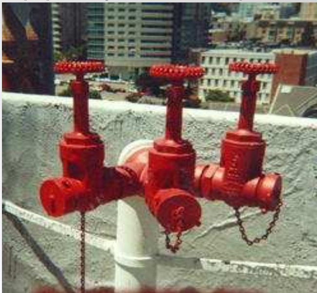
Roof Manifold for Class I Standpipe System Flow Testing
