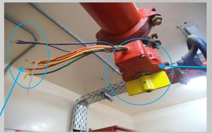
Indicating type butterfly valve with integral supervisory switch
