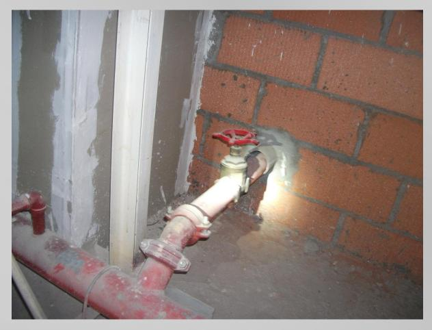
Tenant Isolation Valve for sprinkler system outside tenant boundary line in the Mall's mechanical space.
